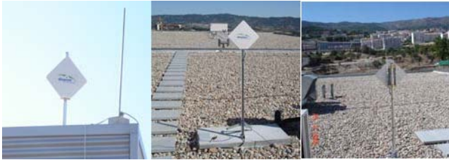
Fig. 7: Pilot BreezeNET B installation.
